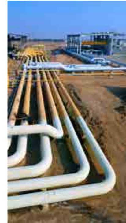
PS-1 Crude Oil Pumping Station Project
